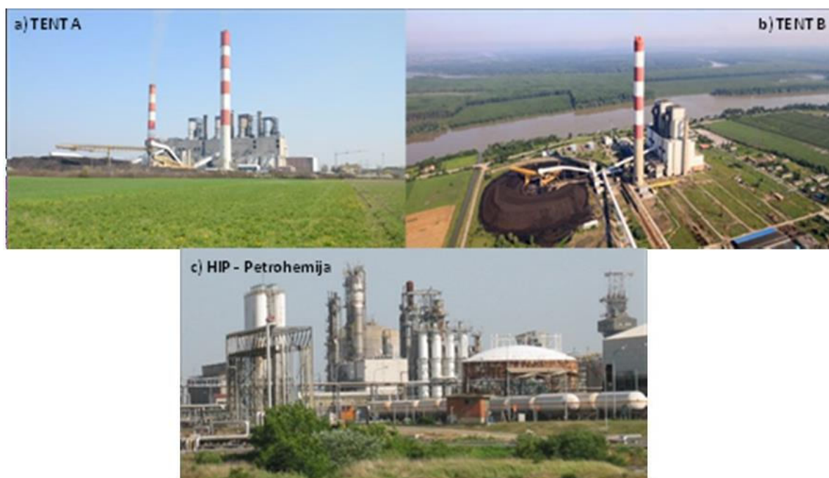
Fig. 1 Republic of Serbia, near Belgrade: Nikola Tesla Thermal Power Plants d.o.o. Obrenovac: Tent A (a) and Tent B (b); industrial-petrochemical complex HIP-Petrohemija a.d. Pančevo (c)
