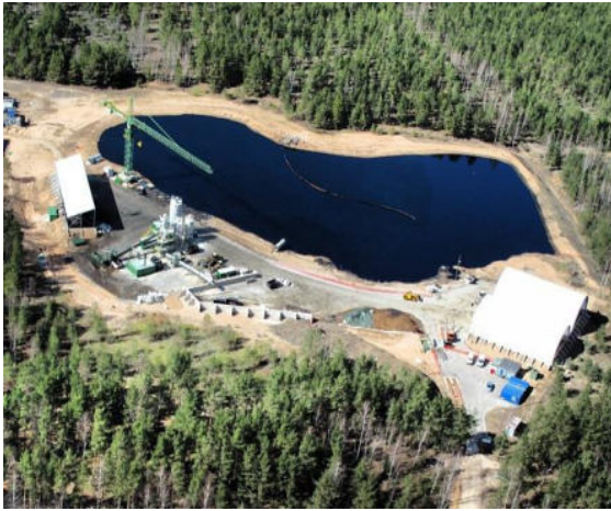
Fig. 2 Remediation of Southern acid tar pond [1]
