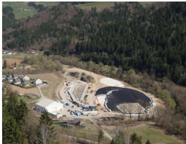
Figure 3. K20 contaminated site (as 28.3.2017) during remediation works
